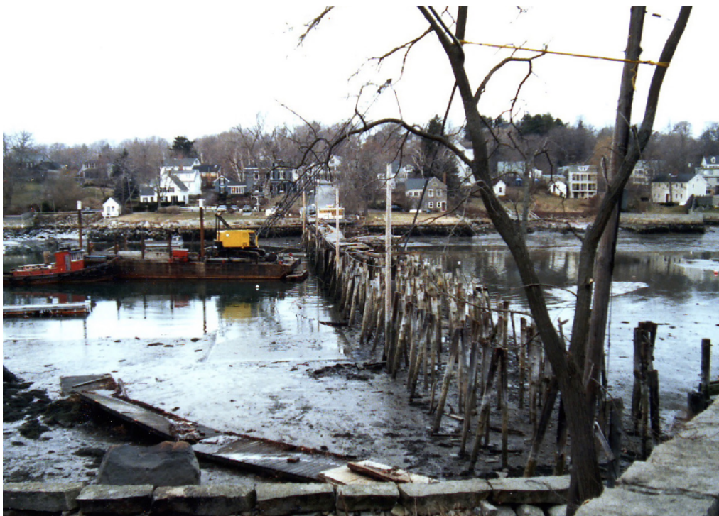
Piles remain after removal of the decking.
